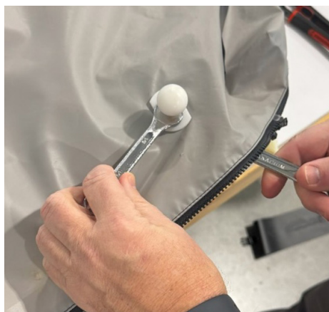
7. Remove the bed footboard anchors with a wrench.
